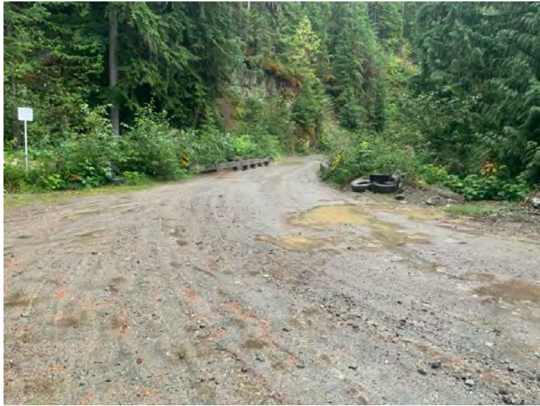
Approach from Right Bank when facing downstream
