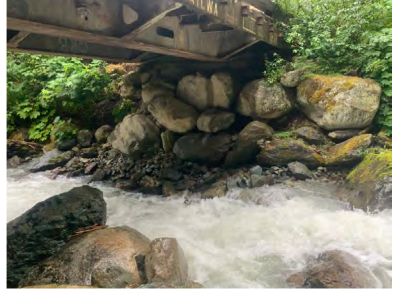
Right Bank Abutment when facing downstream
