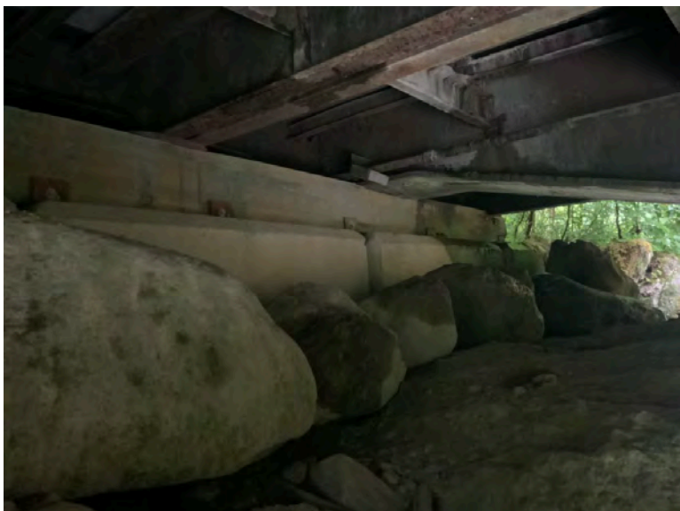
Bearing, right bank
