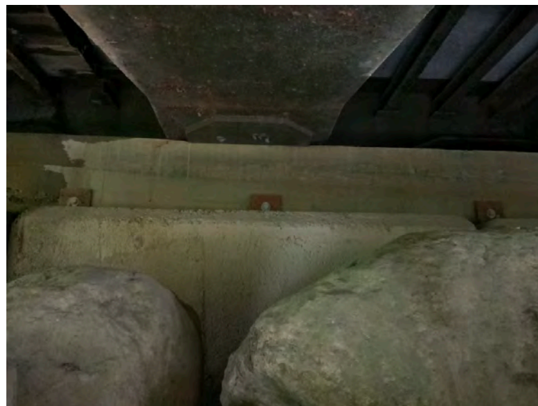
Bearing, right bank
