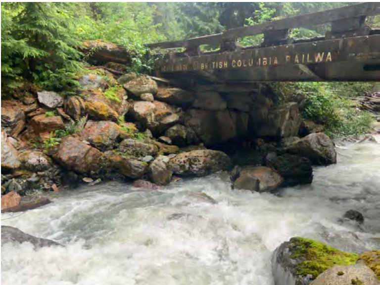
Left Bank Abutment when facing downstream
