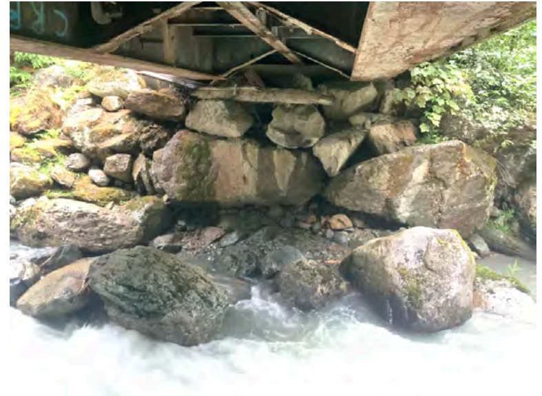
Left Bank Abutment when facing downstream
