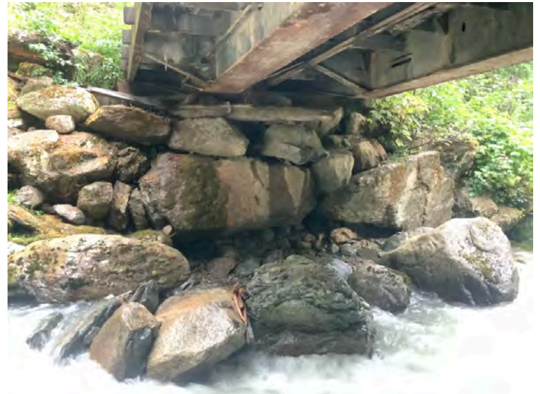
Left Bank Abutment when facing downstream
